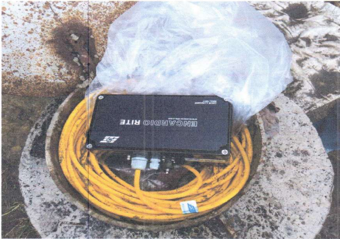
Piezometers (02 Nos.) installed at Rajmahal OCP.
