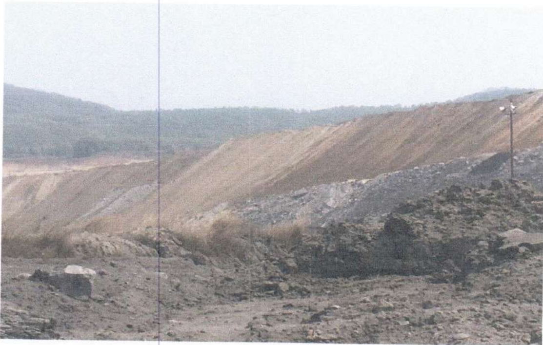
Top Soil Spreading over Technically Reclaimed OB Dumps before Plantation.
