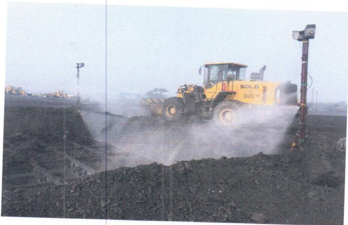
Sensor Based Fine mist water sprinkler at CHP.
