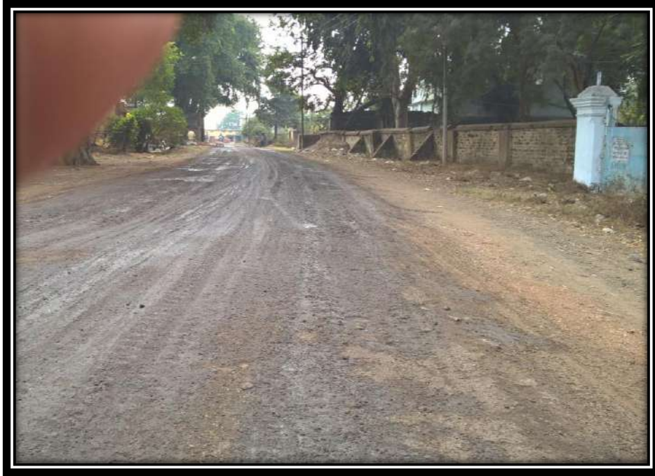
Figure 1 Wet Road after Mobile Water Sprinkling
