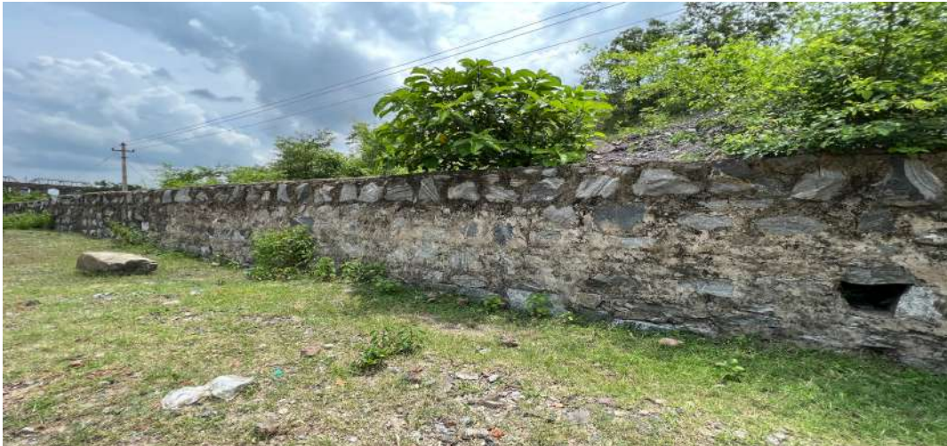
Toe wall around OB Dump
