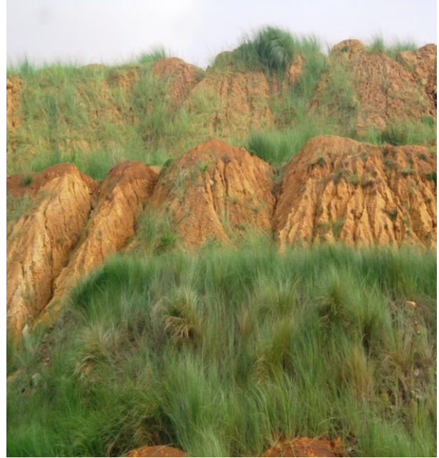
Plate -10: Severely breached external OB dump-D
