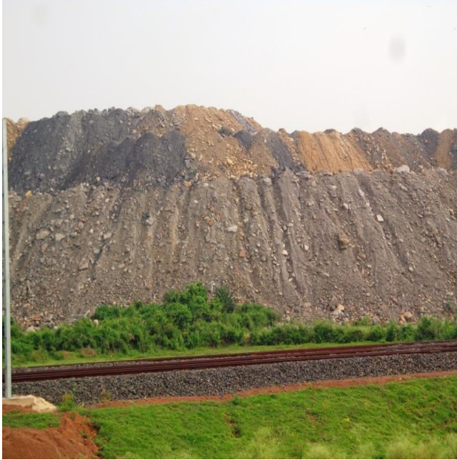
Plate -9: Severely eroded external OB dump- G
