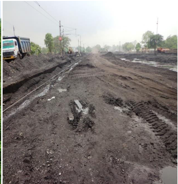
Plate -12: Poorly maintained Sitalpur railway siding
