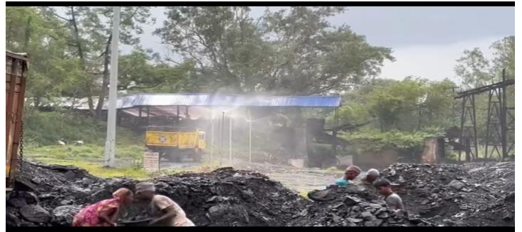
Fixed Water Sprinkling System at Chinakuri Railway Siding.
