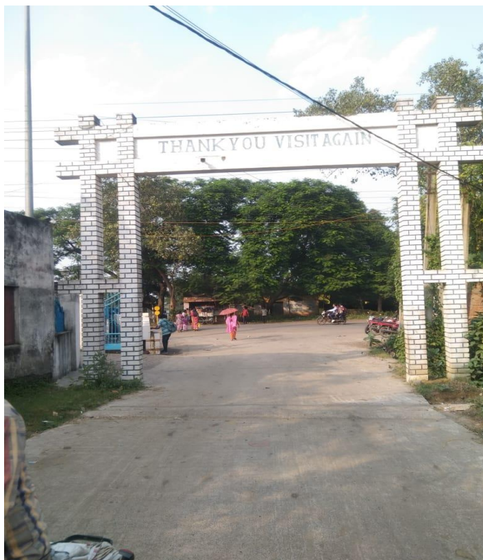
Coal Transporting Road constructed at Dhemomain Colliery
