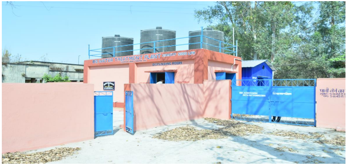
RO PLANT AT CHINAKURI MINE I
