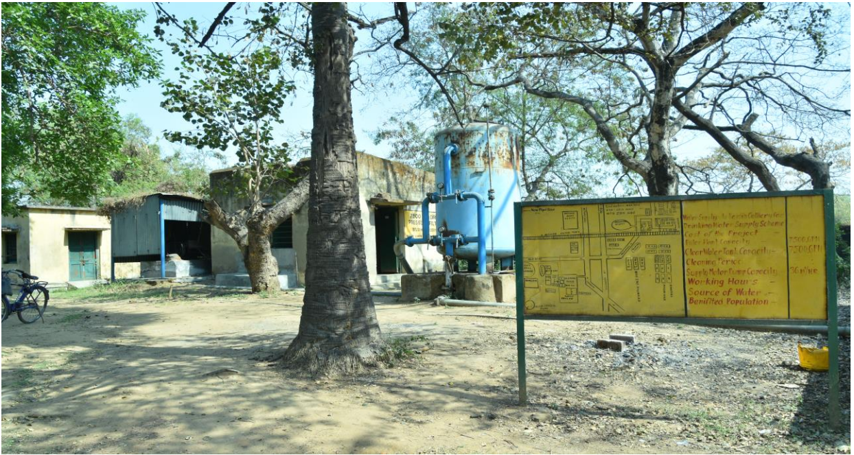
PRESSURE FILTER AT BEJDIH COLLIERY
