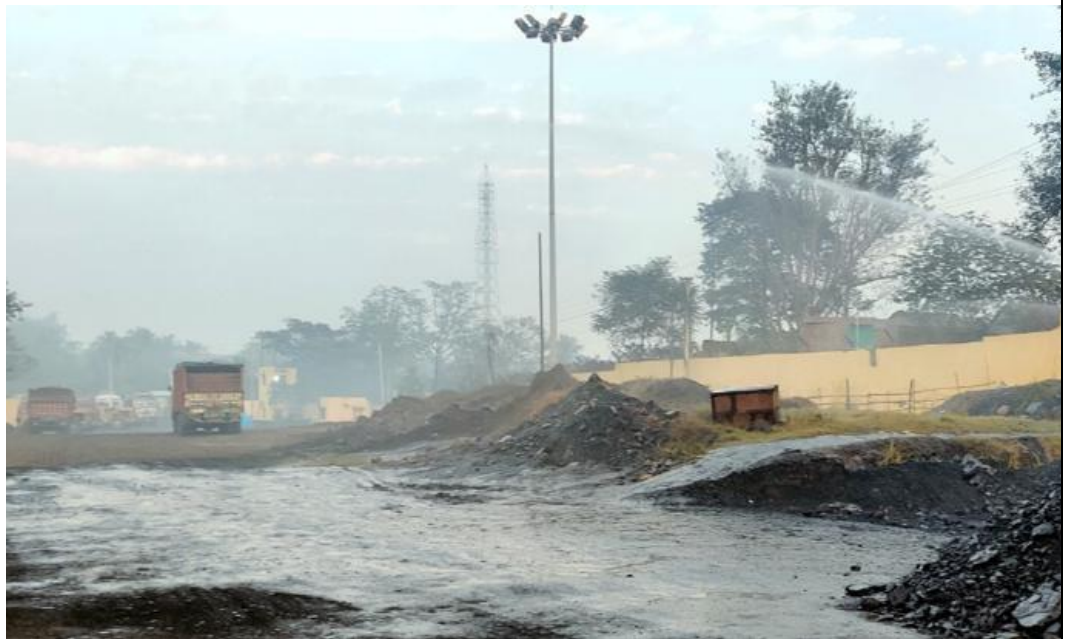
Picture 4: 28 Nos Fixed Type Water Sprinklers at JK Nagar Railway Siding
