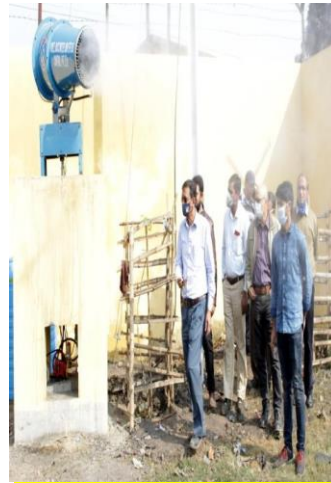
Picture 2: Mist Canon 01 at JK Nagar Railway Siding
