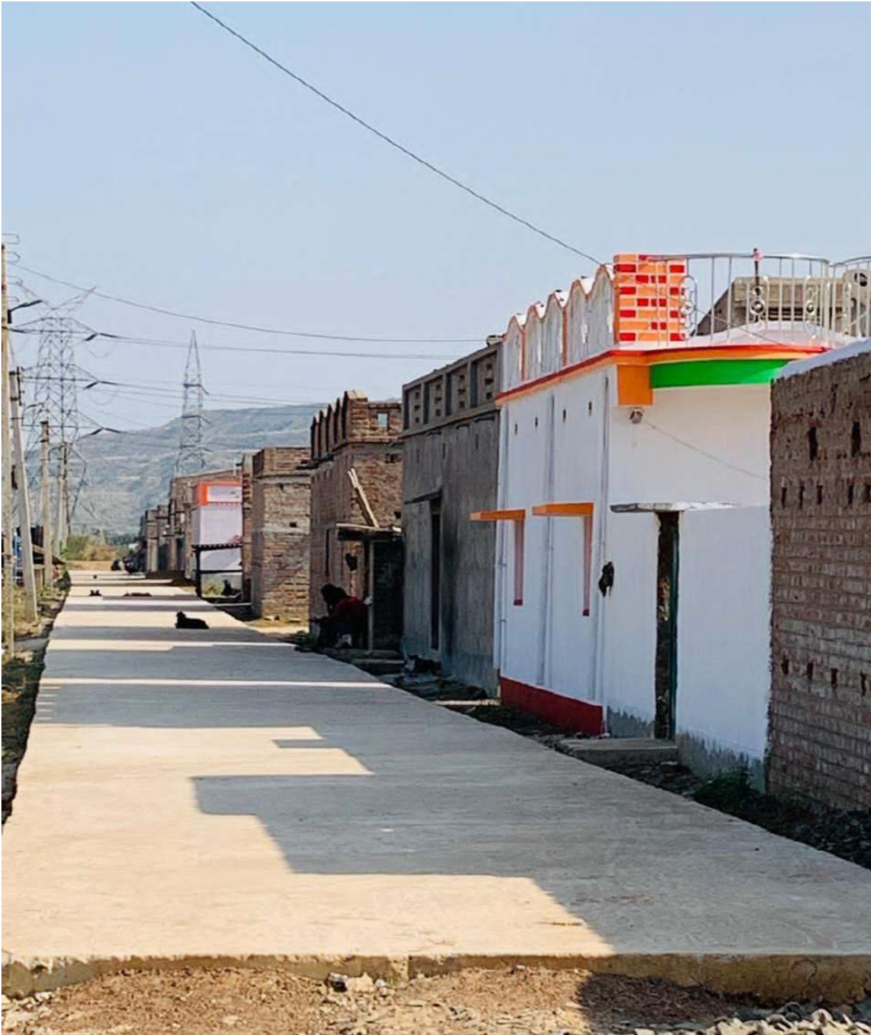
Photograph of constructed house at Bilpahari Rehab Site.
