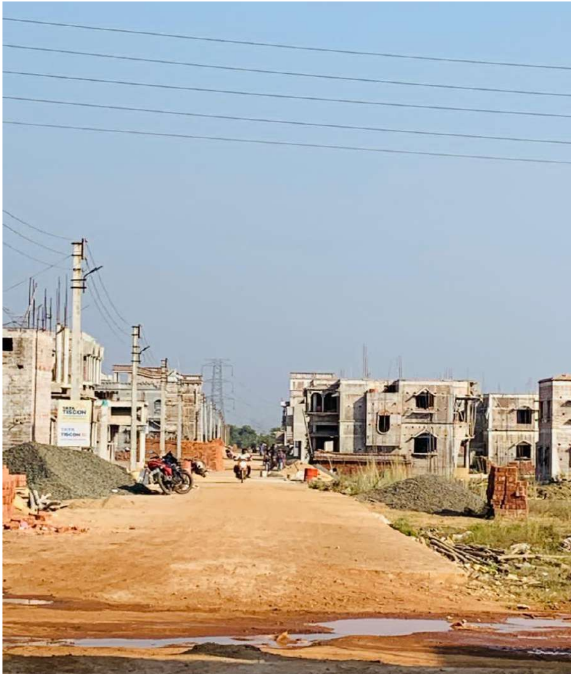
Photograph of under construction houses at Bilpahari Rehab site .
