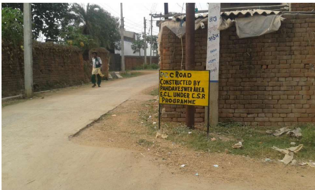
Photograph of PCC road constructed at Madhaipur Village under CSR scheme of ECL
